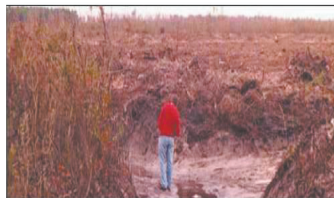
Ditching and draining for pine plantation Green Swamp
