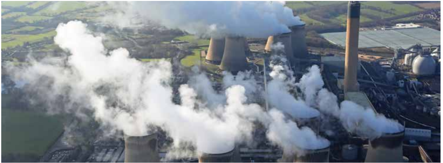
Drax Power Station - North Yorkshire County, England.
